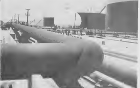
MAZE OF lines carry crude from tankers to agitator tanks and finally back to the tankers that send the product on its way around the world.
